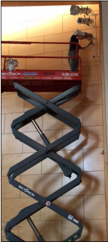
Installing stage lights on high!
