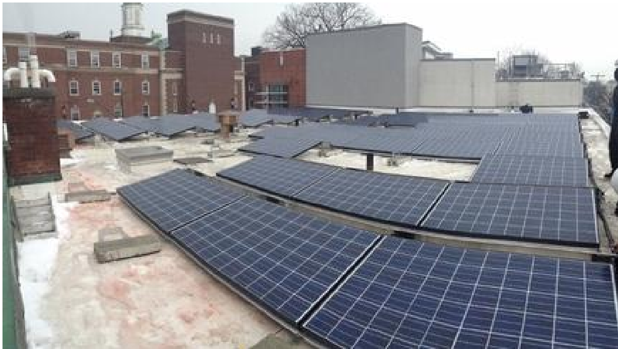
Figure 3: Panels Installed on Our Roof
